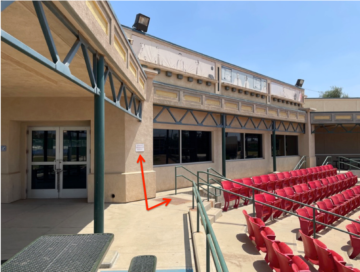
Outdoor seating at the Sportplex adjacent one of the methane sensor vaults and warning signage.
