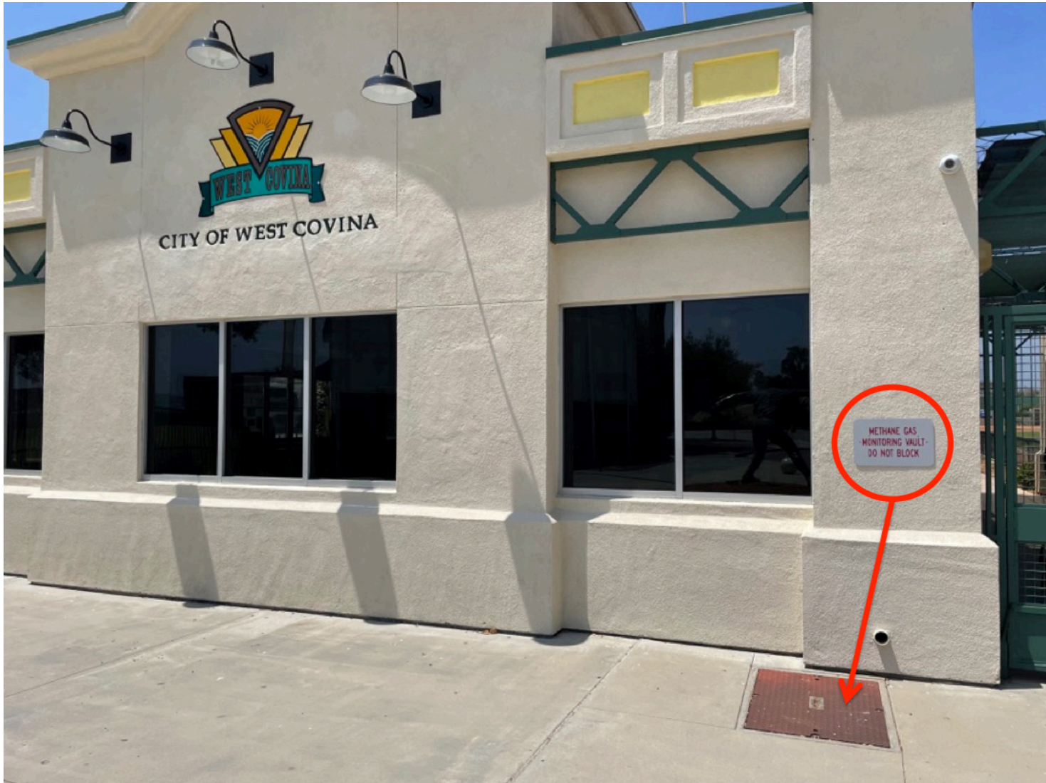
Entrance to the Sportsplex. Sign reads “METHANE GAS MONITORING VAULT DO NOT BLOCK”
